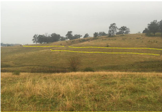
Figure 13 View east showing remnant feeder and irrigation drains curving around the contours from Dam 3 (towards the former dam 4).
